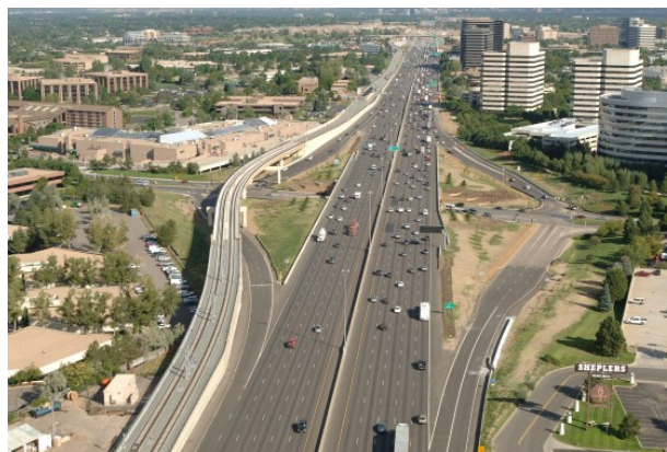
Denver T-REX/ IH 25 Corridor Project — CR in Highway ROW (www.co-asphalt.com)
