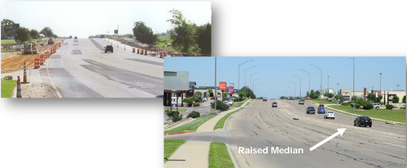
Photographs during construction (2001) of University Drive and after (2012)
