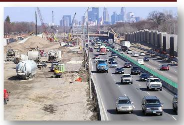
Pavement recycling can significantly reduce construction time and cost by using the existing road structure as part of the new roadway. Breaking up the old pavement and using it as the base material for the final surface lanes (also known as "rubblization" or "full depth reclamation") saves material costs and is much quicker to build.
