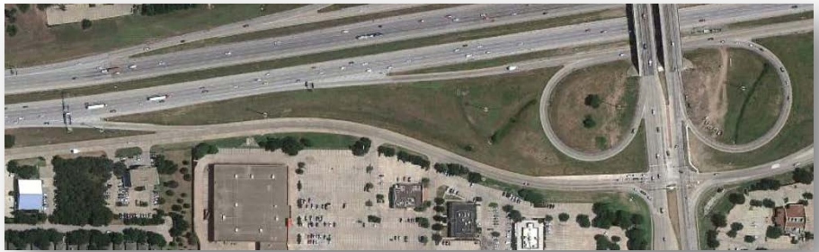
Aerial photograph is of Westbound IH 20 to Southbound FM 157/Cooper Street (initial exit) or Northbound FM 157/Cooper Street (second exit to collector-distributor road and then loop ramp) in Arlington, TX. Source: Google Earth™ Mapping Service.
