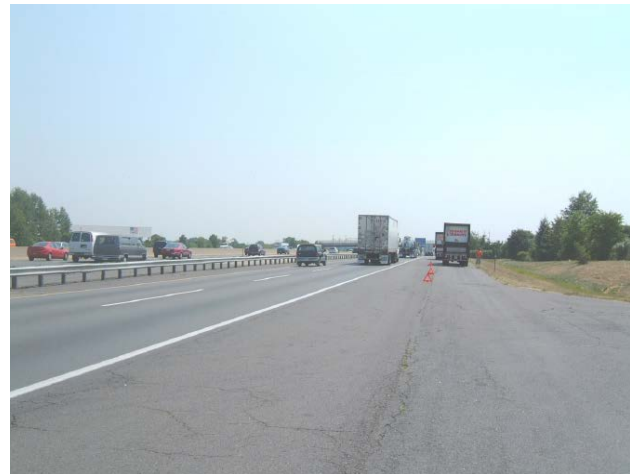
Figure 3. Photo of Extra Wide Paved Shoulder 1
