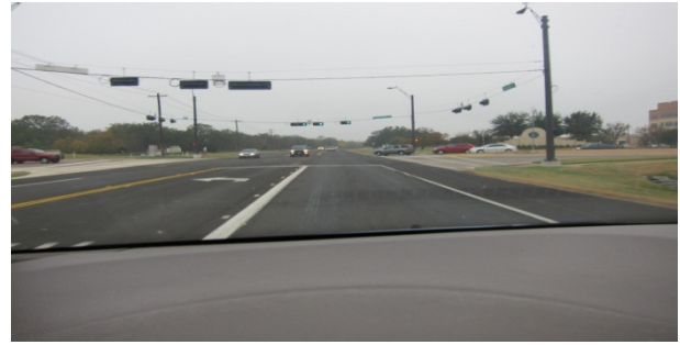
SH 60 After - Left-turn lane installed
