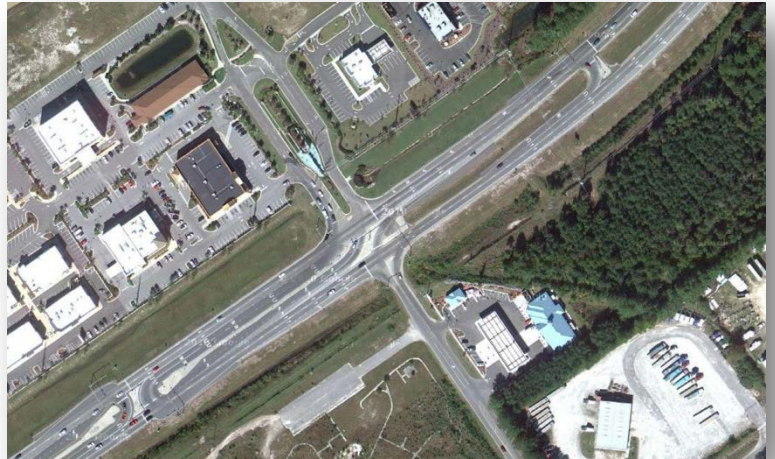
Superstreet with Median U-Turn in Leland, NC (innovativeintersections.org)
